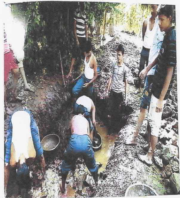
CLEANING THE DRAINAGE AT KATRAL
